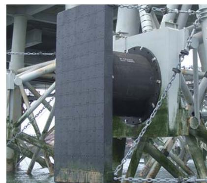
LNG Terminal:Pneumatic Cell ABF-P
